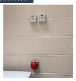
Inside the shower block on the left-hand side wall are 2 fixed fuse switches. The two illuminated ones side-by-side heat the water in the copper tank. As a rule they are normally left on; if they are off, switch them back on.
